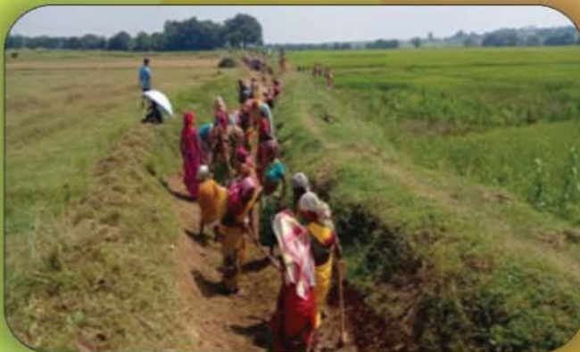
Cannel renovation under DFW
